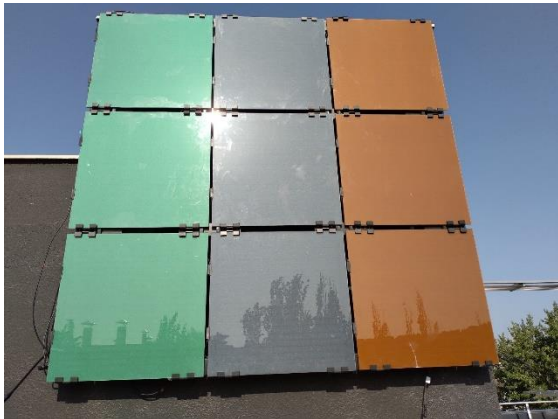
Figure 3: Colored ventilated façade developed in the project at CIEMAT.
